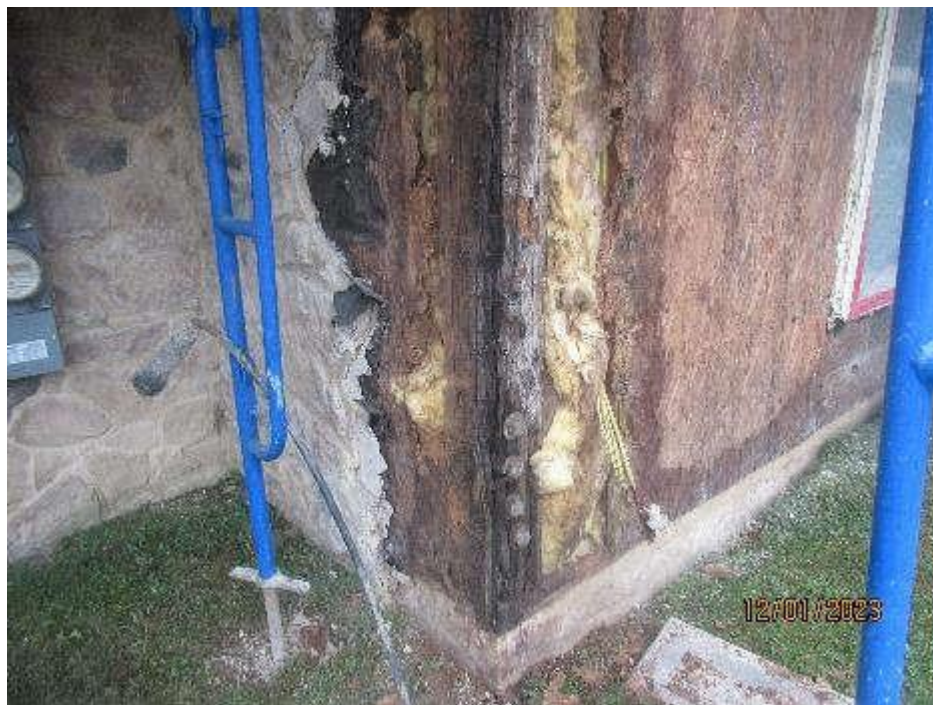
Unit 216 North Elevation – PSL Column has been replaced at the corner by the CMU wall.
