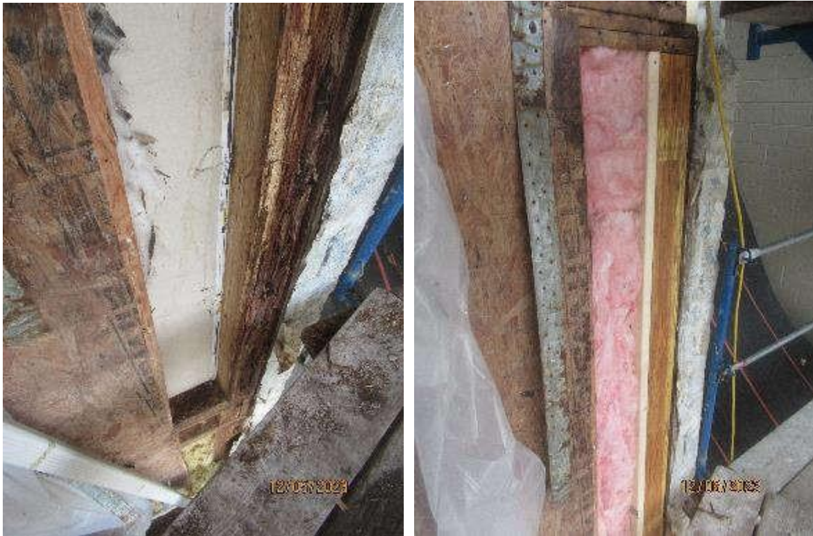
Unit 216 North Elevation – PSL Column has been replaced at the corner by the CMU wall.
