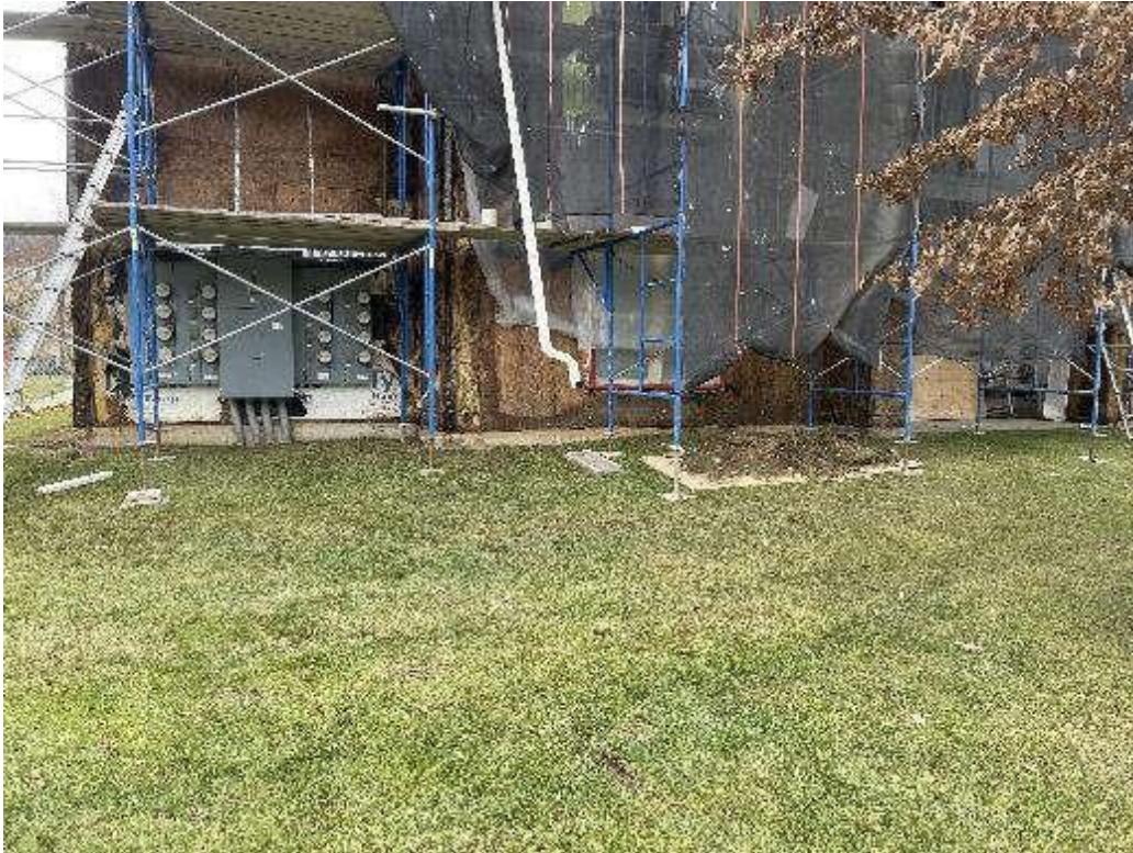
Northeast Side of Building 3000 – Foundation is above grade. No Foundation Waterproofing required.
