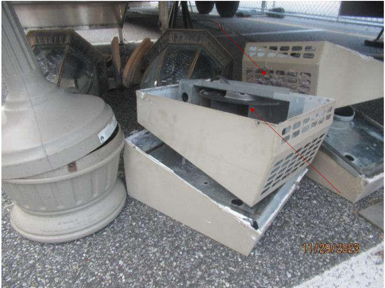
Existing dryer vent cover with built in powered fan. Existing dryer vent cover showing trapped lint.
