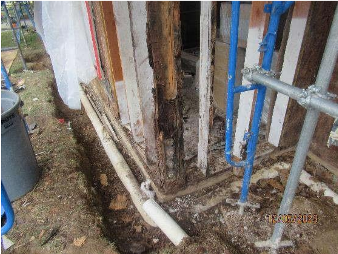
Unit 115 North Elevation – Damage at the outside corner at the West side of the unit.
